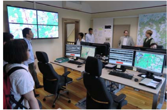
A forest fire surveillance centre
