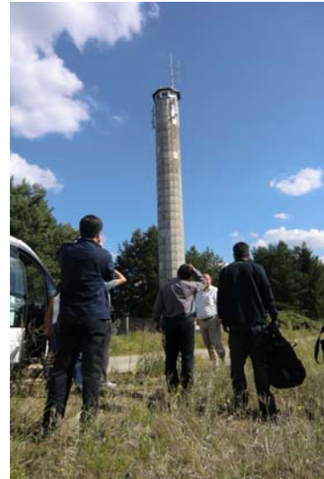
Fire protection tower for the early detection and localising of fires
